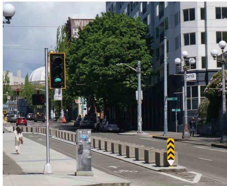
Seattle's Pike Street Bridge was re-channelized and the sidewalks widened to provide enhanced bicycle and pedestrian facilities.
